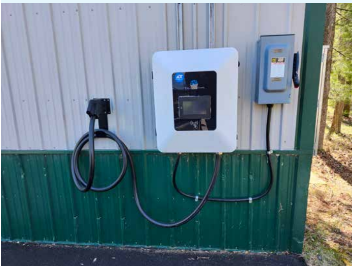
Figure 10. Level 2 EV charging station at the Mille Lacs Band of Ojibwe Department of Natural Resources office. Photo from Charlie Lippert, Mille Lacs Band of Ojibwe
